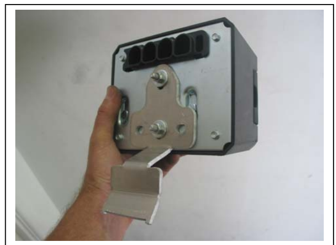
Figure 6: control box mount installed
